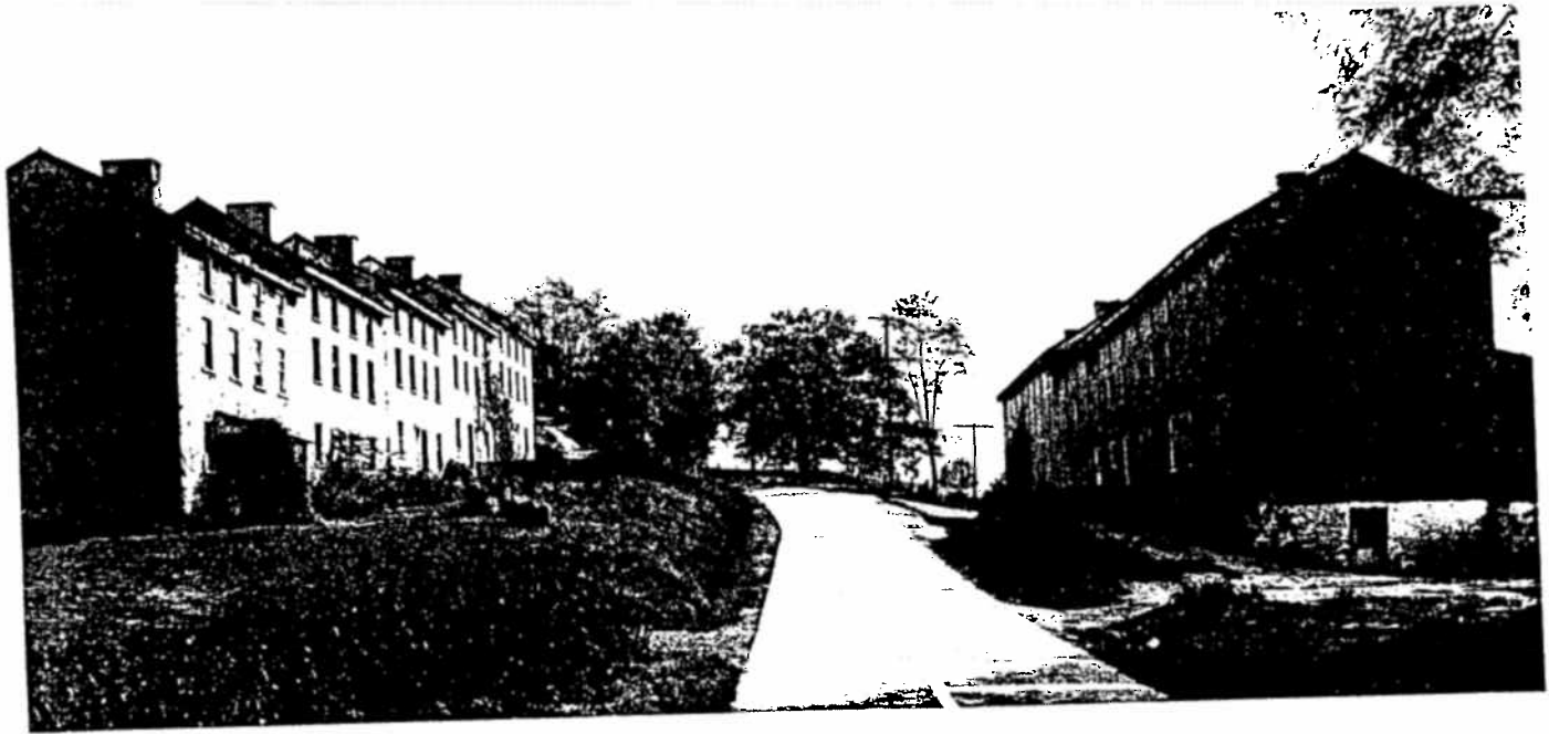
CE-163 & 164, Elk Forge tenements (1936, Historic American Buildings Survey)
